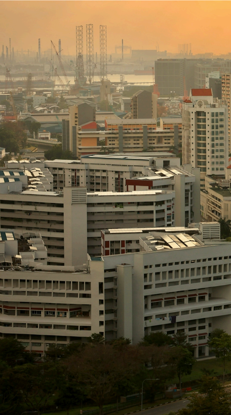
Solar PV installations on the rooftops of HDB blocks in Singapore.
